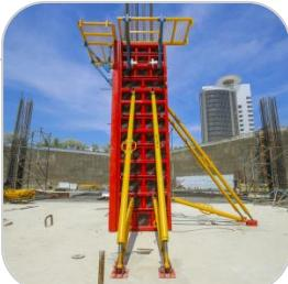
**Houpad Formwork Wall, Slab, and Column...**
